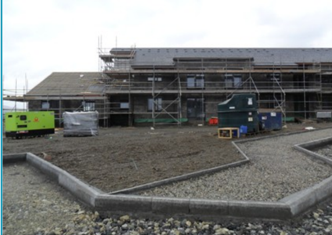
Mull Progressive Care Centre under construction
